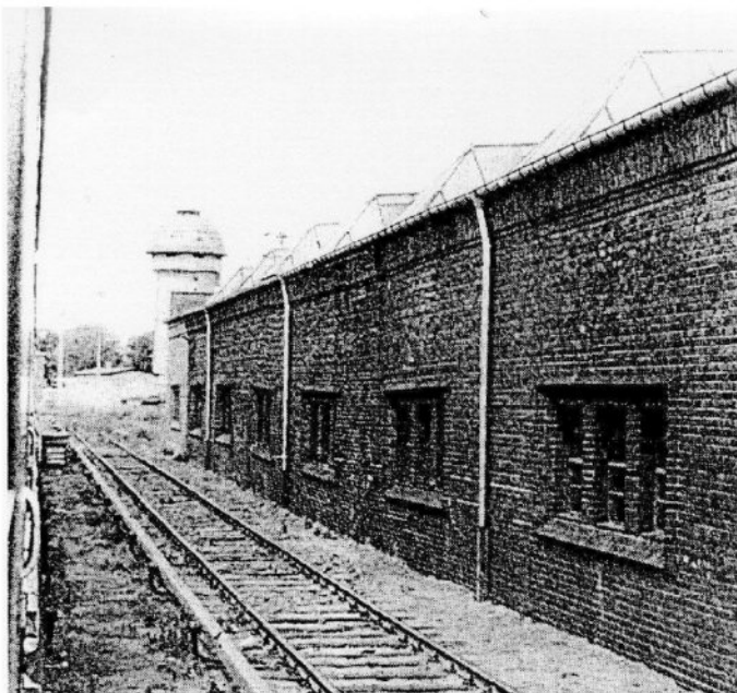
Figure 2: Building near a "S-Bahn railway"
