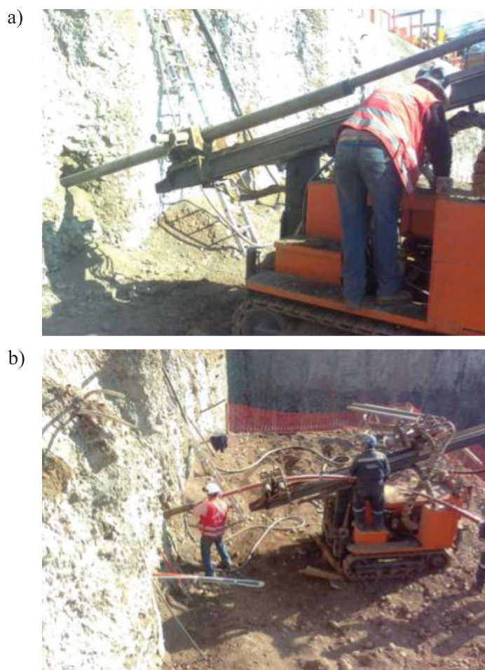
Figure 6: Installation of Energy Anchors: a) ground drilling, and b) cable and HDPE pipes are inserted.
