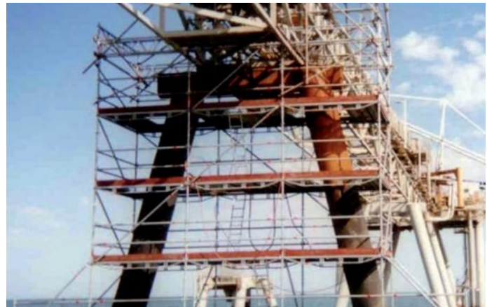
Figure 1: Bridge piles under corrosion control and maintenance.
