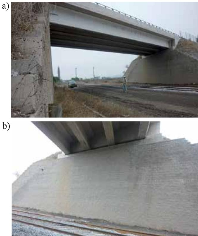
Figure 2: a) View of the motorway bridge Las Gaviotas over railway and road and b) view of the geogrid reinforced soil wall abutment
