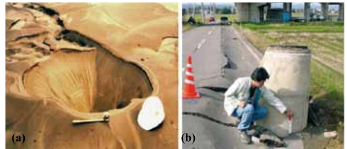
Figure 2:a) Sand boil, Loma Prieta earthquake 1979 (USGS 2006) and b) manhole uplift Niigata ken-Chuetsu earthquake 2004 (GEER 2004)
